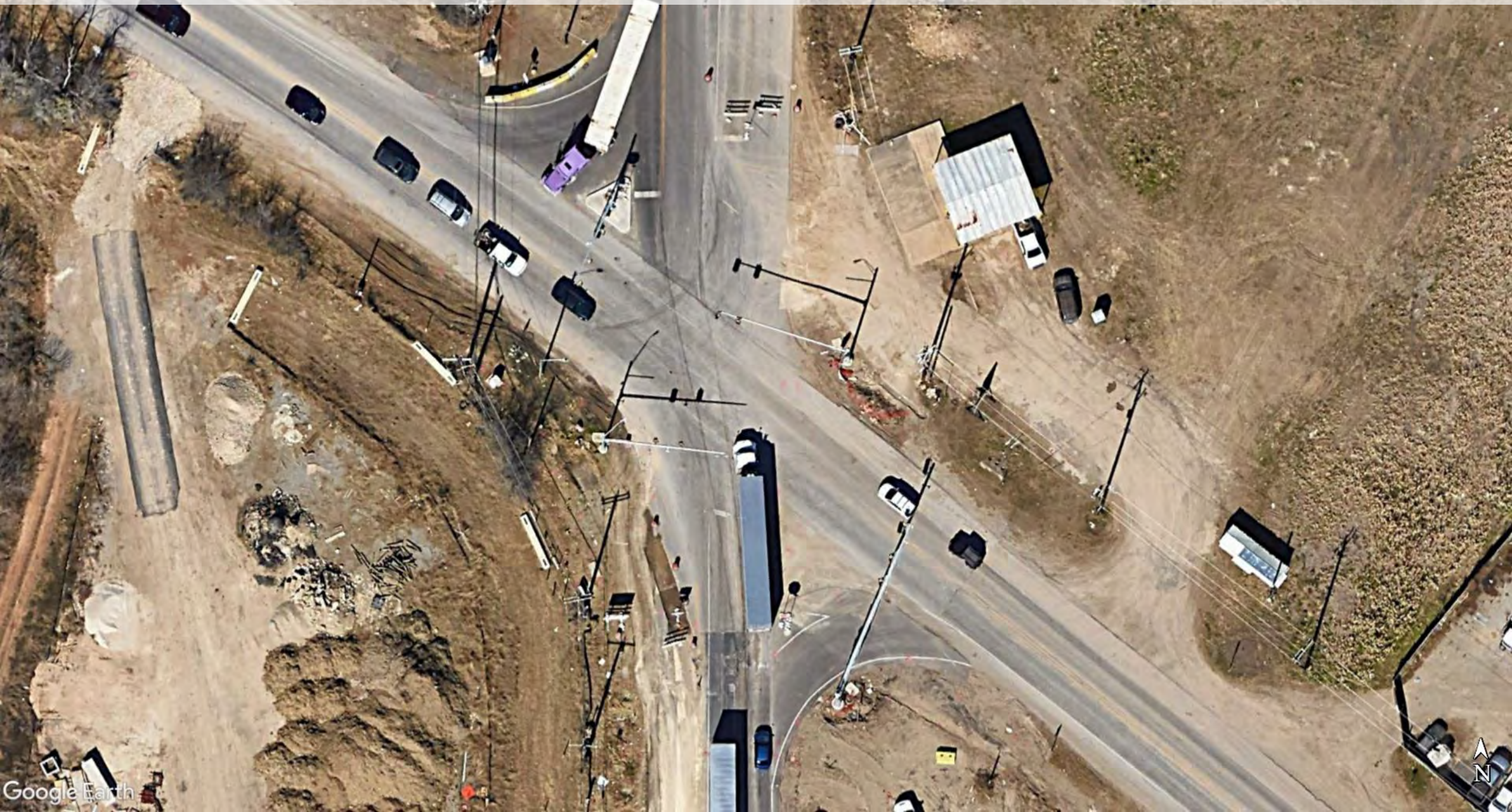
Figure 36: Mobility Site C - East Houston Street and South Foster Road - Existing
