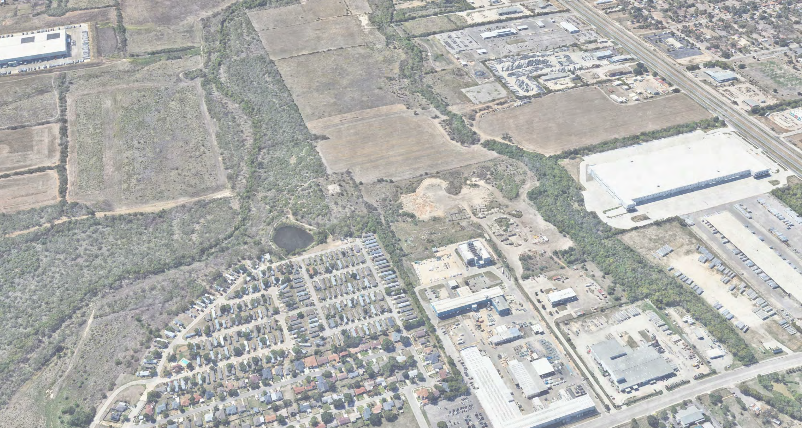
Figure 24: Transformative Project: East Loop 410 – Existing (Looking South)
